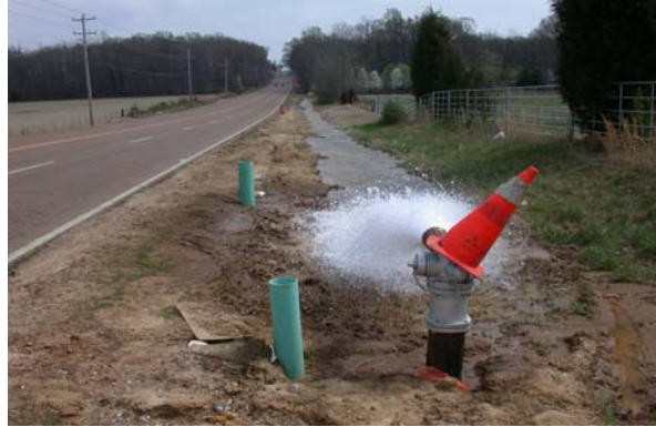
Water line construction near Lakeland City Hall (March 2004)
