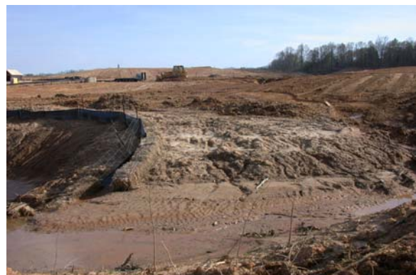
Filling of flood plain (March 2004)
