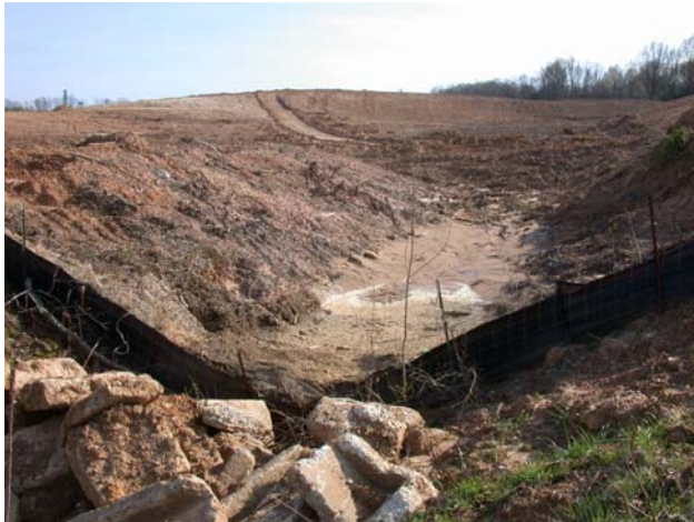
Construction along Oliver Creek (March 2004)
