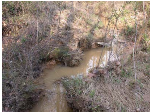
Same tributary downstream of construction. Muddy flow on dry day (sample location 02) (March 2004)
