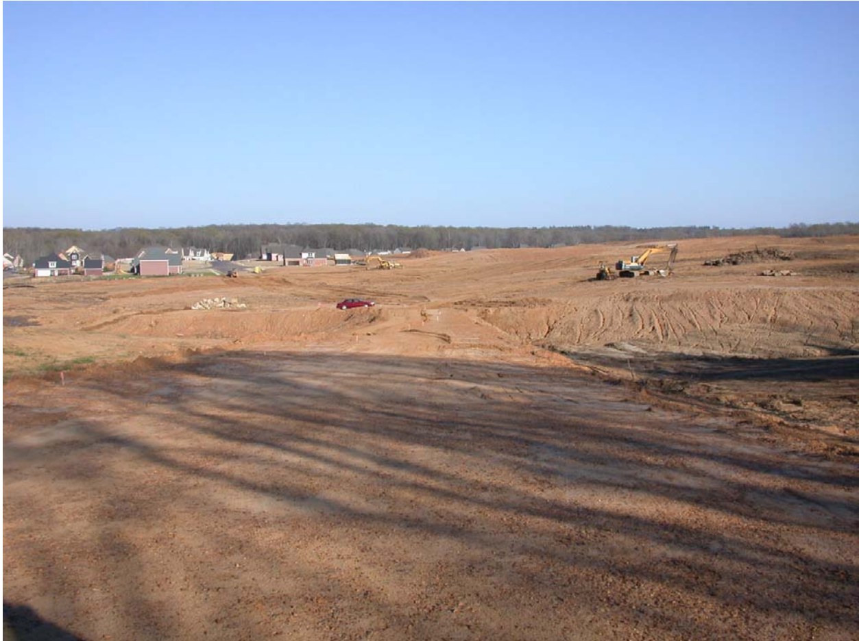
Massive flood plain development along Oliver Creek (background trees) with no sediment controls visible. (March 2004)
