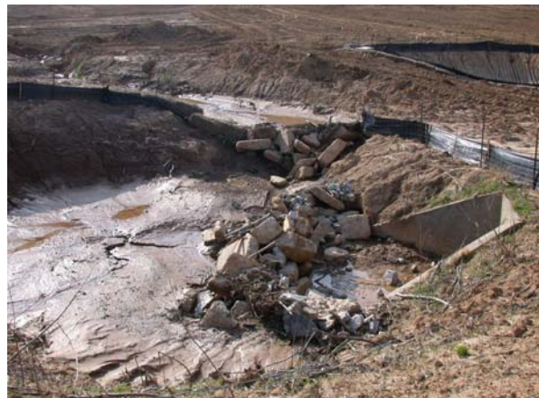
Construction in tributary to Oliver Creek (March 2004)
