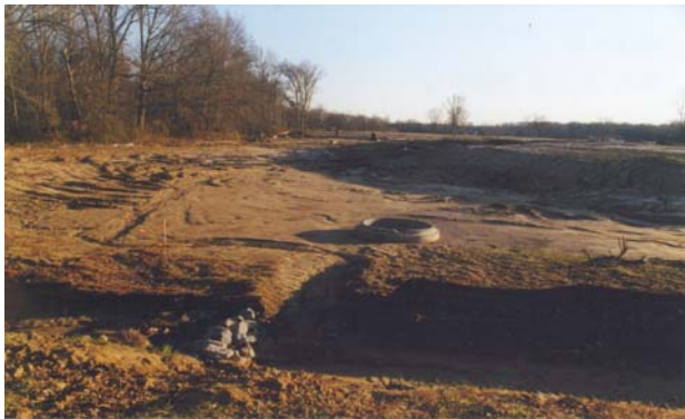
Filling of flood plain at Oliver Creek (December 1999)
